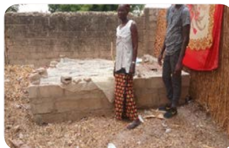
Compost pit built in Thiak, filled and protected to accelerate maturation
