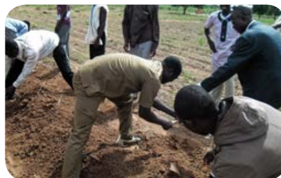
Construction of earth embankments
